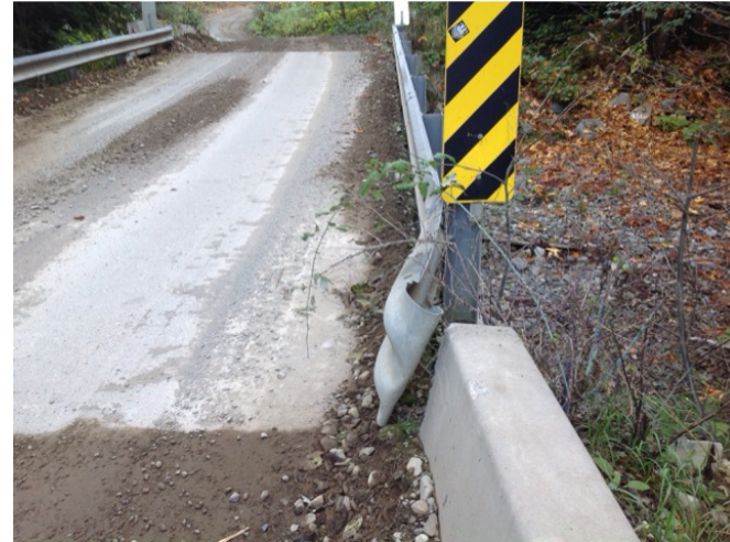
guardrail damage
