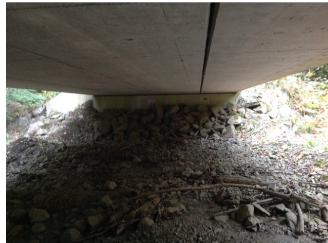
Right Bank Abutment when facing downstream
