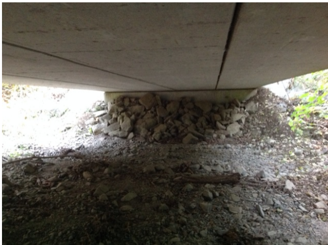
Left Bank Abutment when facing downstream
